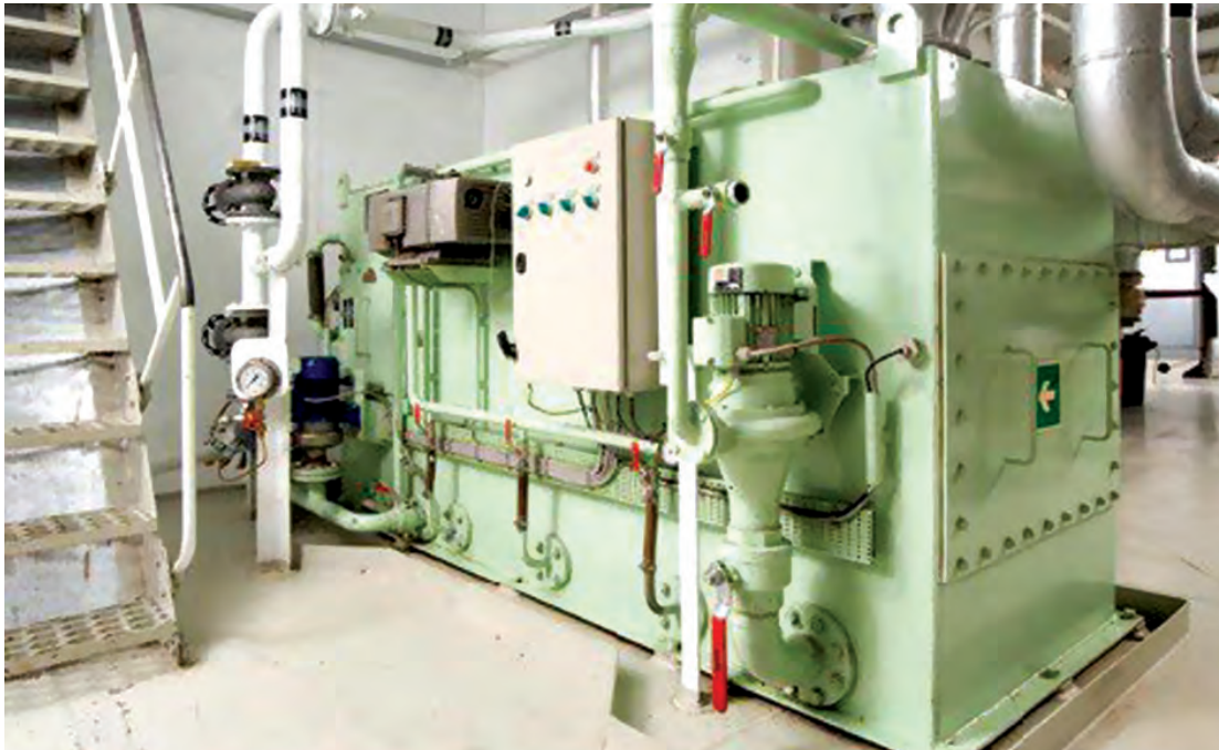
sewage treatment plant
