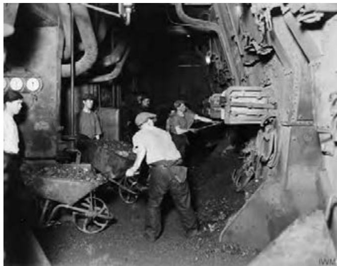
Steam ships boiler room
