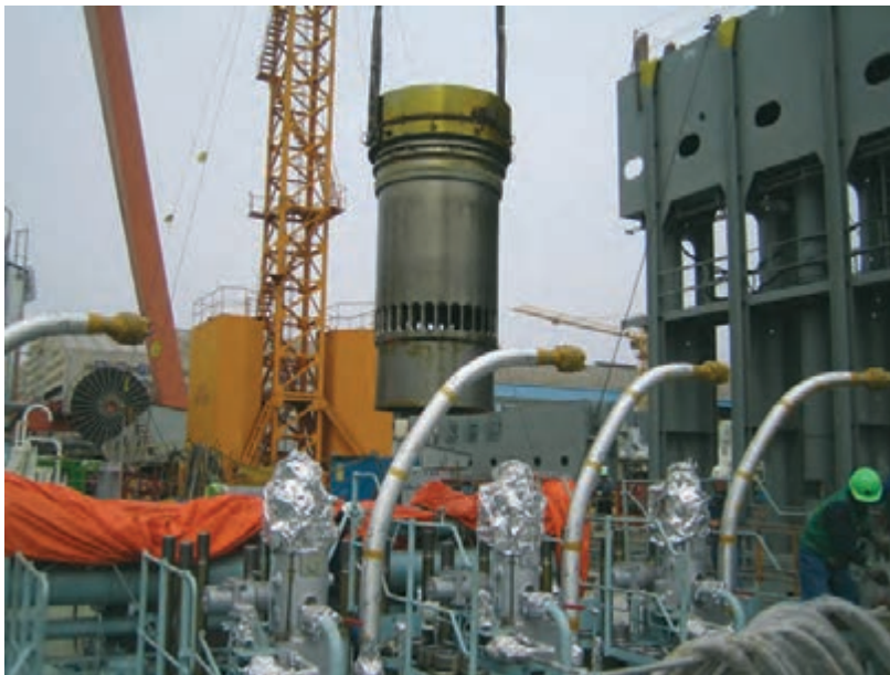
Fig 27: Big engine cylinder liner
