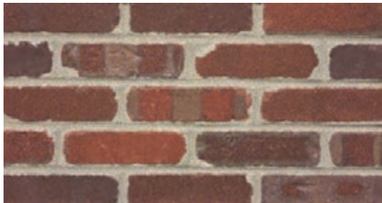
Standard 3/8" Mortar Joint
