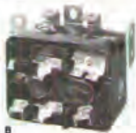
Figure 8-61. Potential starting relay. A—With casing removed, components are visible. Weight (1) closes the points (3) during the off cycle. On starting, increasing voltage into the coil (2) will pull contact points apart and stop current flow through the starting winding. B—A similar potential relay with casing in place. (White-Rodgers Division, Emerson Electric Co.)
